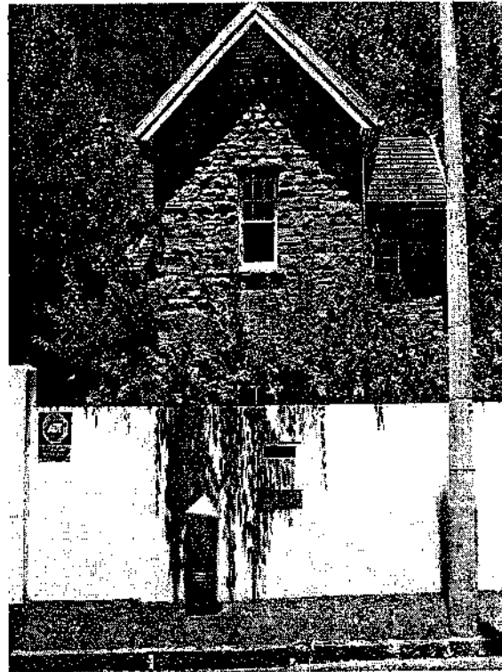
Figure 2.16 Access taken from side street
