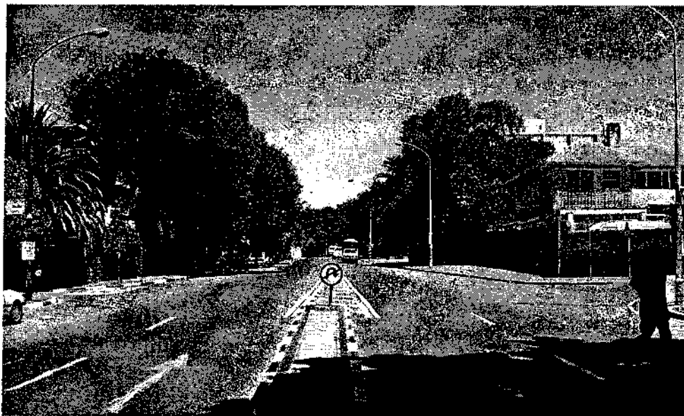
Figure 2.2 Double carriageway gives way to single carriageway
